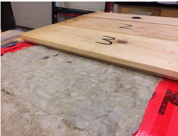
Photograph 3: View of partially installed pine siding boards.
