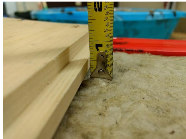
Photograph 4: View clear airspace between pine siding boards and mineral fibre insulation.
